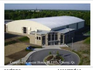
CURVED ROOF STEEL BUILDING is ideal for projects requiring clear spans up to 80 meters (262 feet) depending on the region. They are a cost-effective solution for construction of arenas, indoor soccer fields, gymnasiums and applications requiring column -free space
